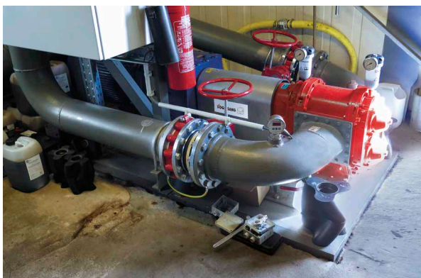
The VX186-260 QD rotary lobe pump pumps the molasses from the jetty to the storage tank on the shore.
