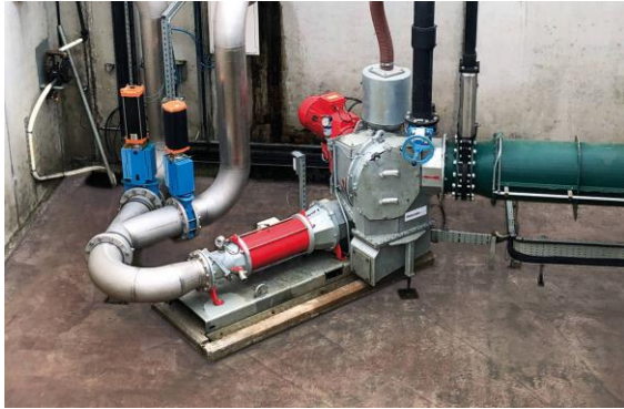
Image 1: The universal PreMix solid matter feeder mashes different substrates into a homogeneous organic suspension.
